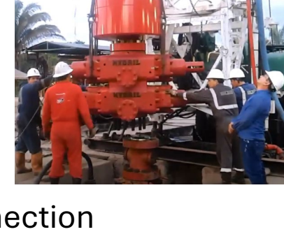
Installing casing head
