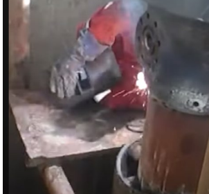
welding casing head
