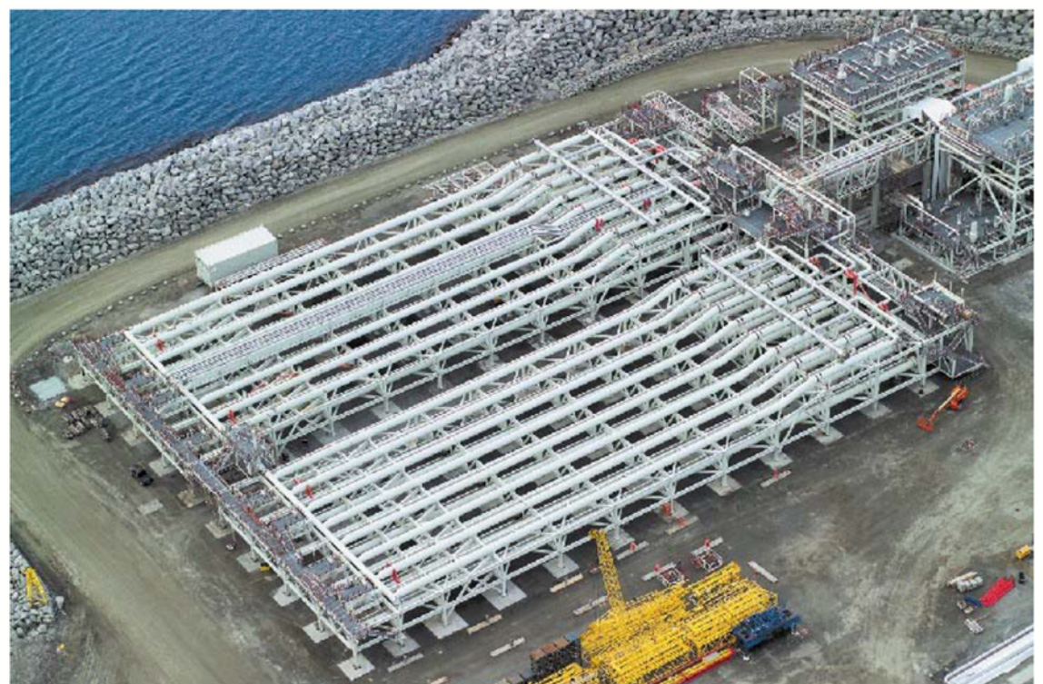
Slugcatcher – link between offshore and onshore systems
