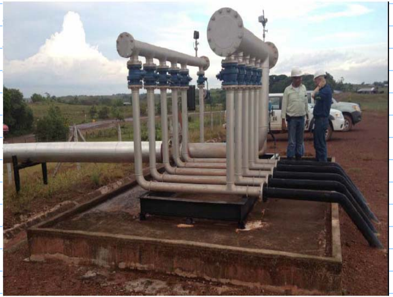
field in Colombia, production manifold and liquid flow meter
