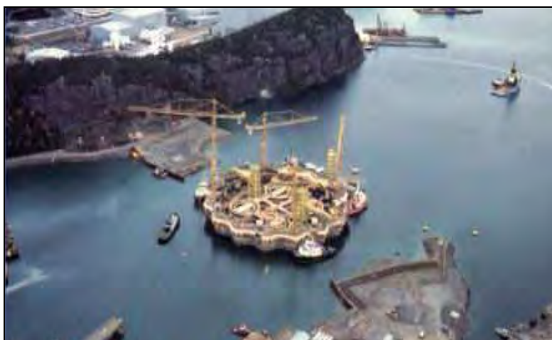
Figure 10.4-2: Hibernia GBS Leaving Dry Dock
