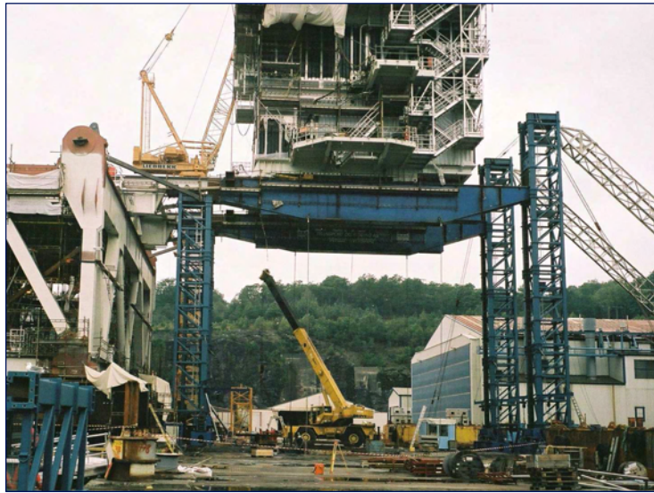
Figure 10.4-5: Example of Module lifted by use of Lifting Towers
