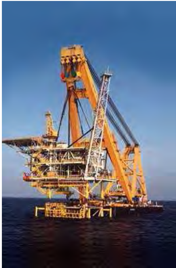
Figure 10.4-6: Example of Floating Shear Leg Installing a Complete Topsides
