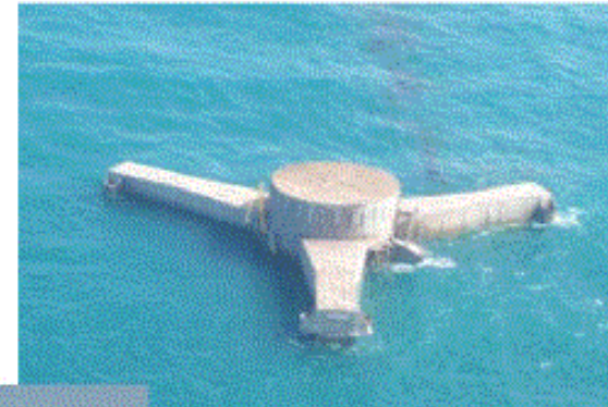
Typhoon upside down after hurricane Rita
