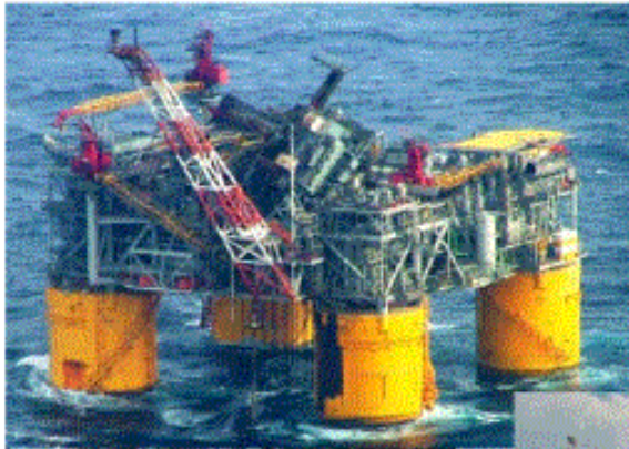
The Mars TLP after the hurricane Katrina
