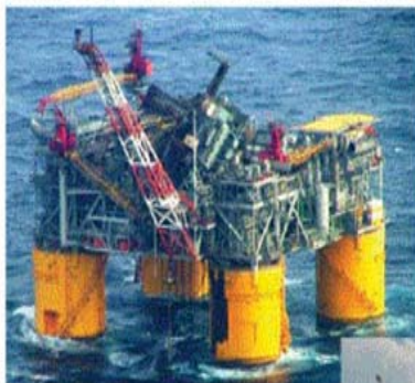
The Mars TLP after the hurricane Katrina
