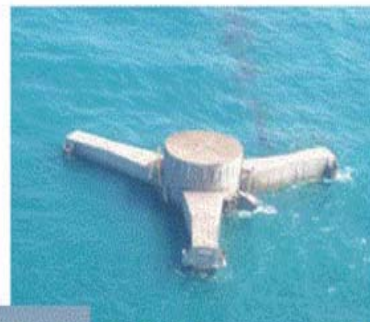
Typhoon upside down after hurricane Rita
