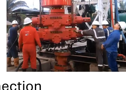
Installing casing head
