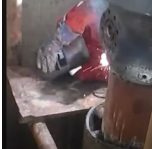
welding casing head
