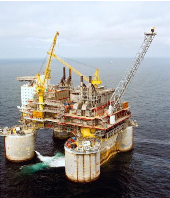
Figure 1: The concrete floating production platform, Troll B.
