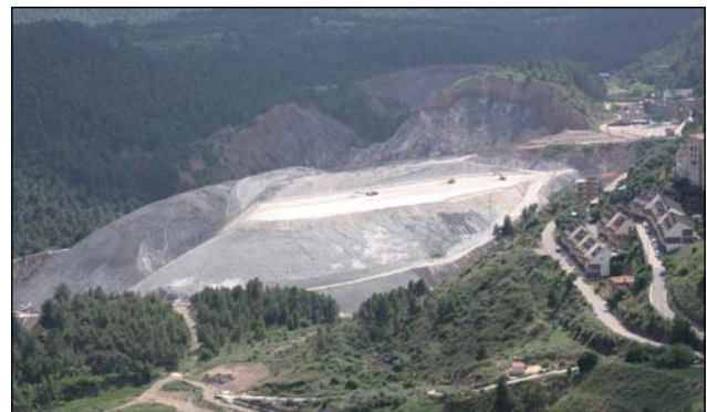
Figure 1 The Cardona salt diapir outcropping just behind the large body of salt dump. To the right, part of the town of Cardona, is the ancient shaft and the entrance for visitors. The salt is flanked by reddish lacustrine-fluviatile sequences, and capped by brownish Quaternary sediments.
