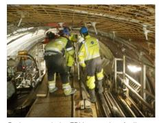
Rock support during TBM-excavation of railway tunnel (Ulriken, Bergen).
