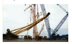
Uprighting a trusswork section for a steel jacket platform.
